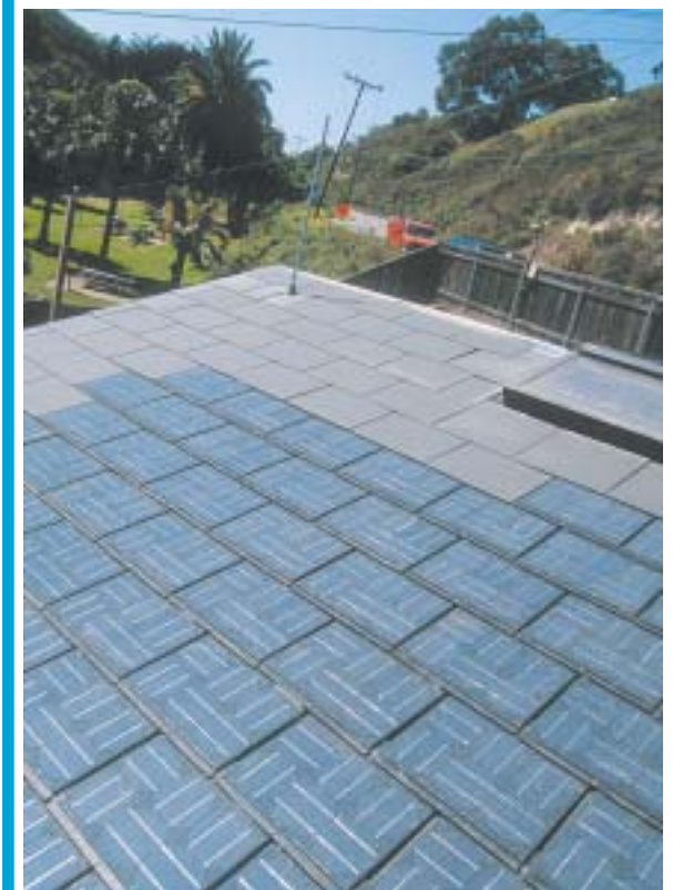
These solar tiles line the roof at the Watershed Resource Center at Arroyo Burro Beach.
